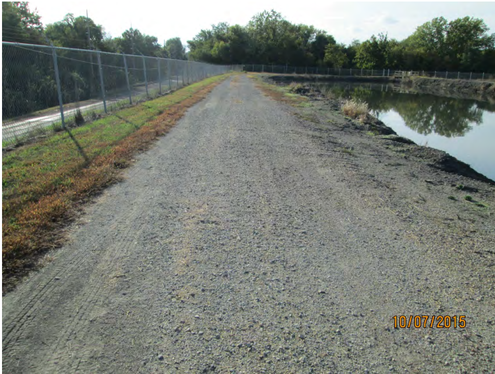
Photo No. 5 South Berm Crest
