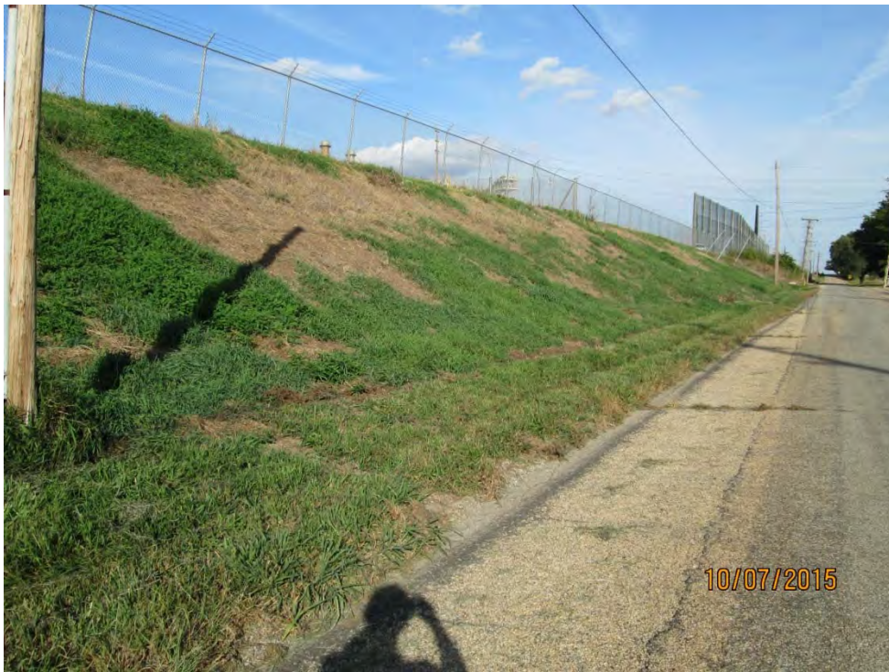
Photo No. 14 South Downstream Slope
