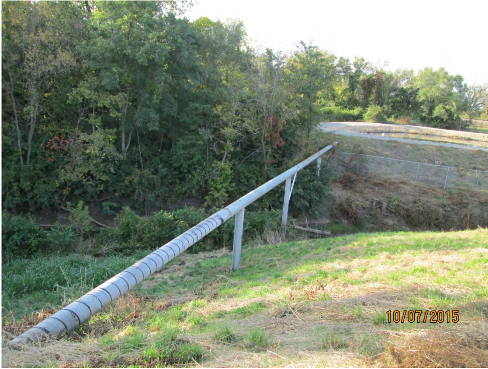
Photo No. 23 Outflow Pipe
