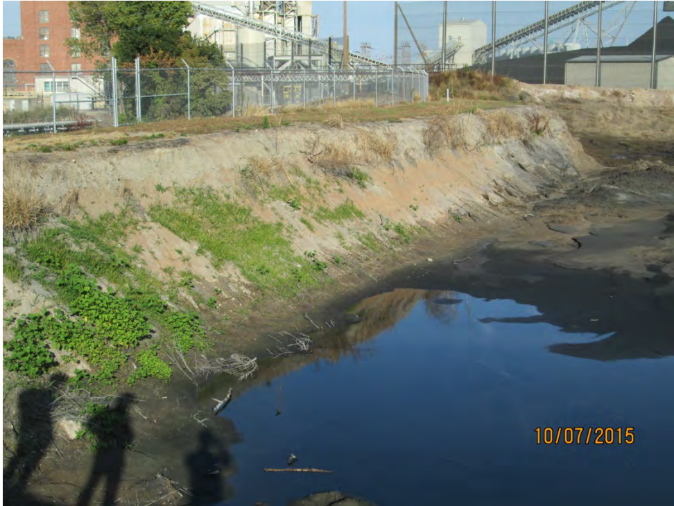
Photo No. 9 North Berm Upstream Slope
