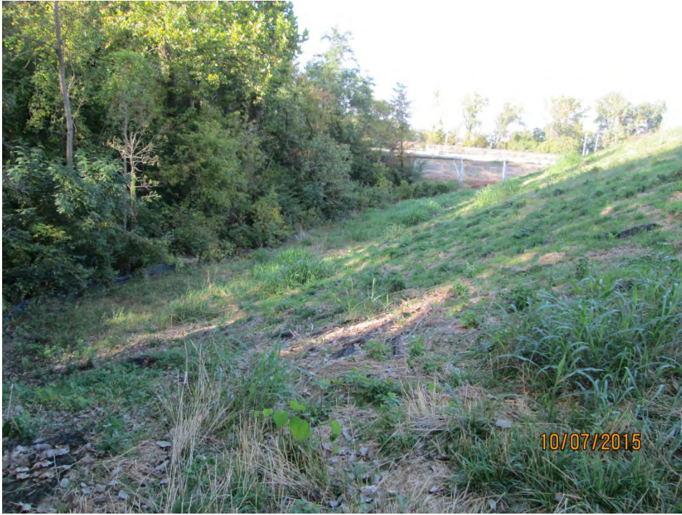
Photo No. 11 West Berm Downstream Slope
