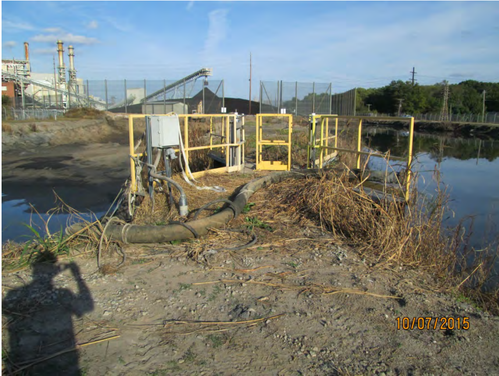
Photo No. 21 Intake Structure
