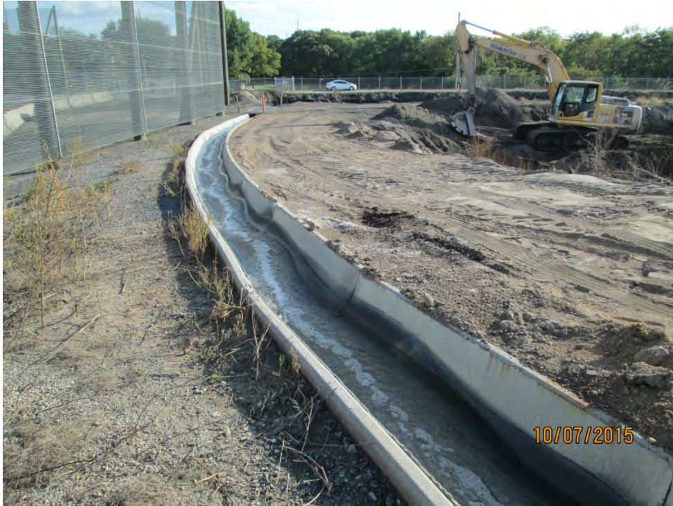
Photo No. 25 Inlet Channel to South Pond
