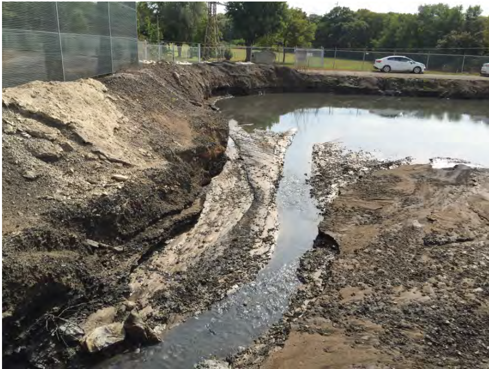
Photo No. 26 Discharge from Inlet Channel into South Pond
