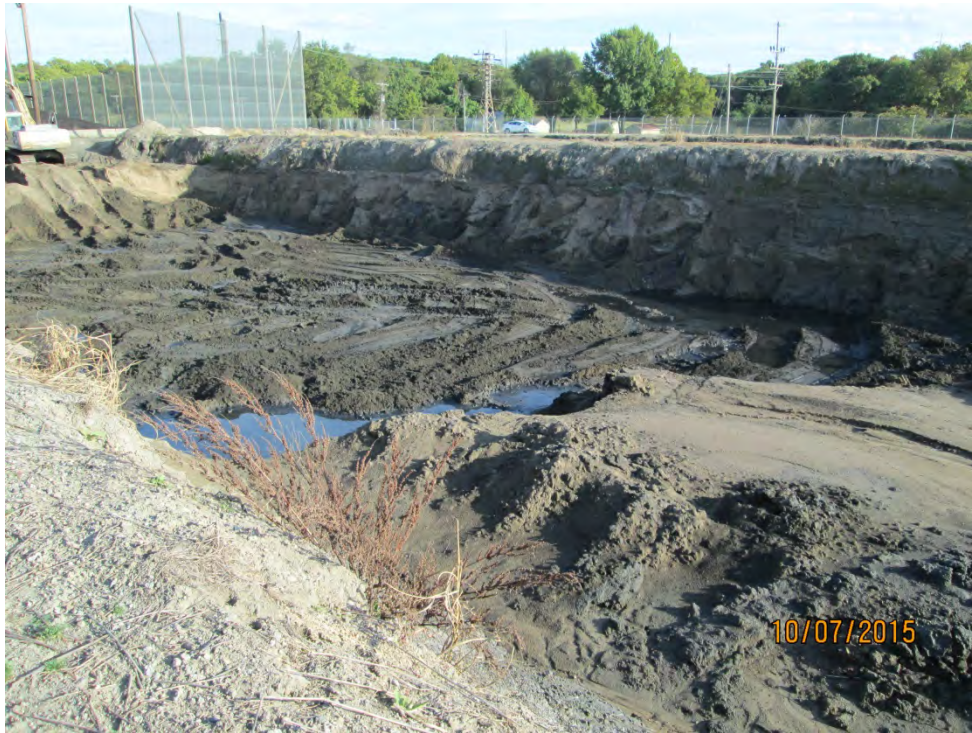
Photo No. 4 North Pond – Area of Ash Removal
