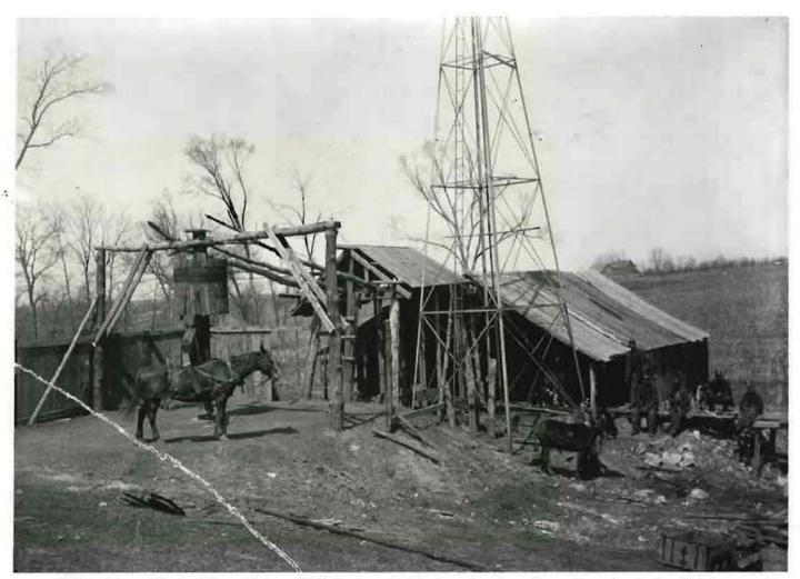
James Brothers Mine at Bevier, Missouri (circa 1911). The horse hoisted coal and supplies up the mine shaft, which is covered by the sheds. The mine car in the right foreground was used underground to haul coal from the working face to the main shaft.
