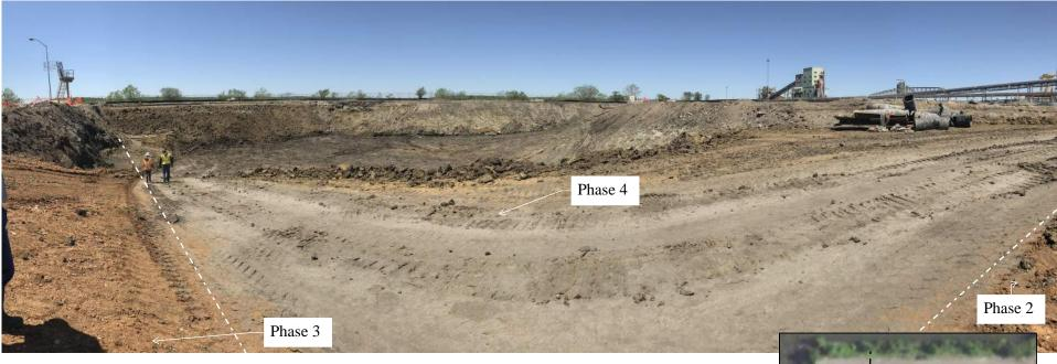
Photo was taken on May 8, 2020, at a centrally-located point from within the Impoundment, looking north/ north-east, at the completion of CCR removal. Backfill of the Phase 3 area can be seen to the west of the viewpoint. Clay was observed at the base of the unit. Survey information for this phase was taken on May 8, 2020.
