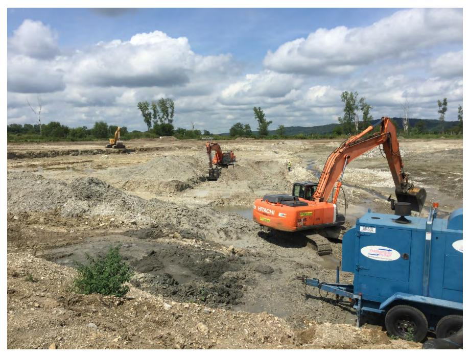
Figure 3: Iatan Ash Impoundment – mechanical excavation from north portion of pond (looking northeast)
