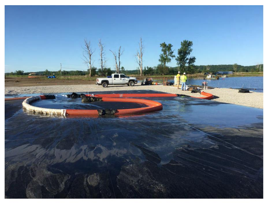
Figure 10: Iatan Ash Impoundment – installing geotextile tube system (east bank looking south)
