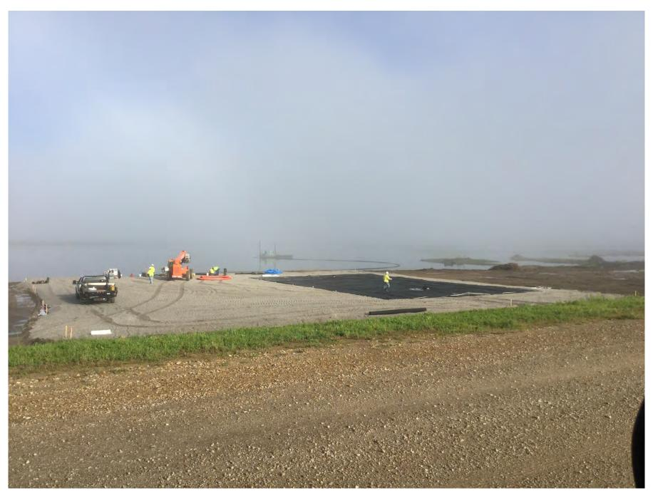
Figure 9: Iatan Ash Impoundment – prepping geotextile tube area (east bank looking west)
