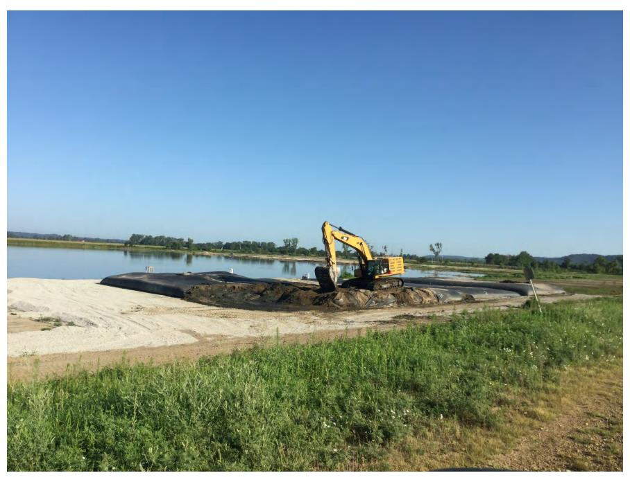
Figure 14: Iatan Ash Impoundment – excavating ash from geotextile tubes (east bank looking northwest)
