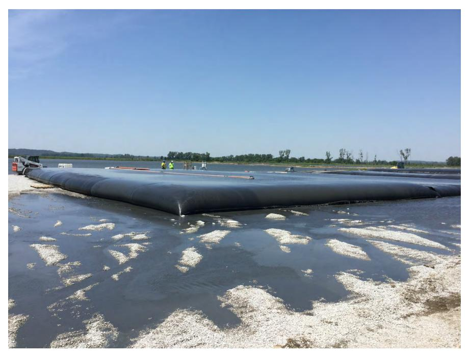
Figure 12: Iatan Ash Impoundment – filling geotextile tubes (east bank looking northwest)
