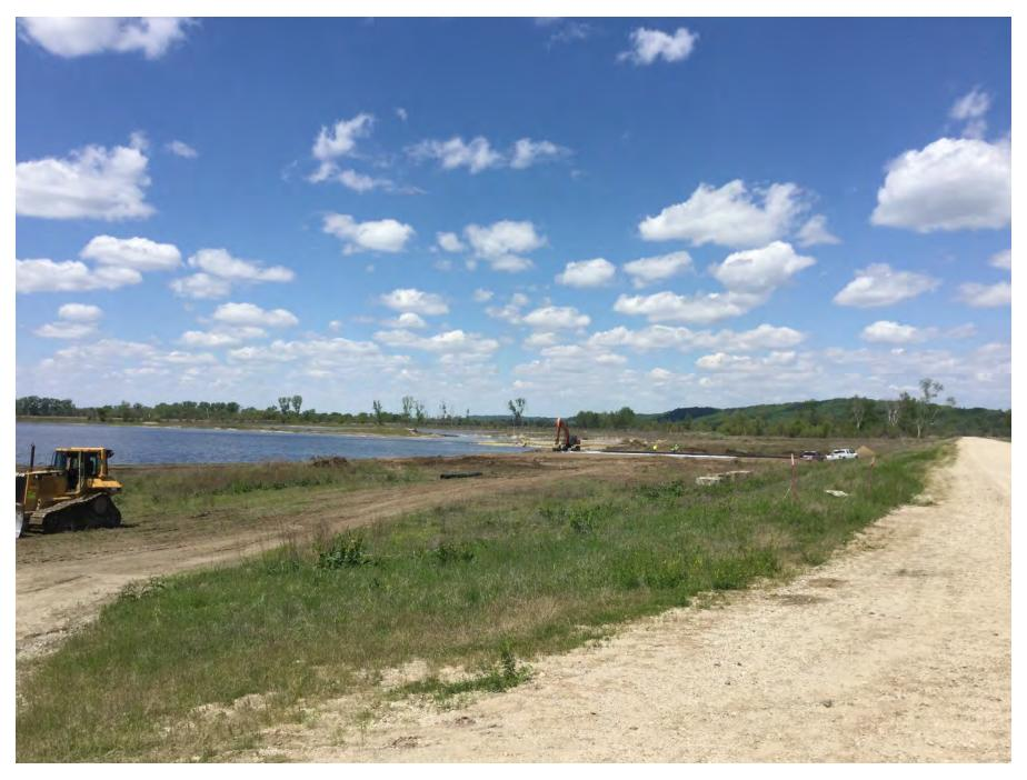
Figure 8: Iatan Ash Impoundment – prepping geotextile tube area (east bank looking north)
