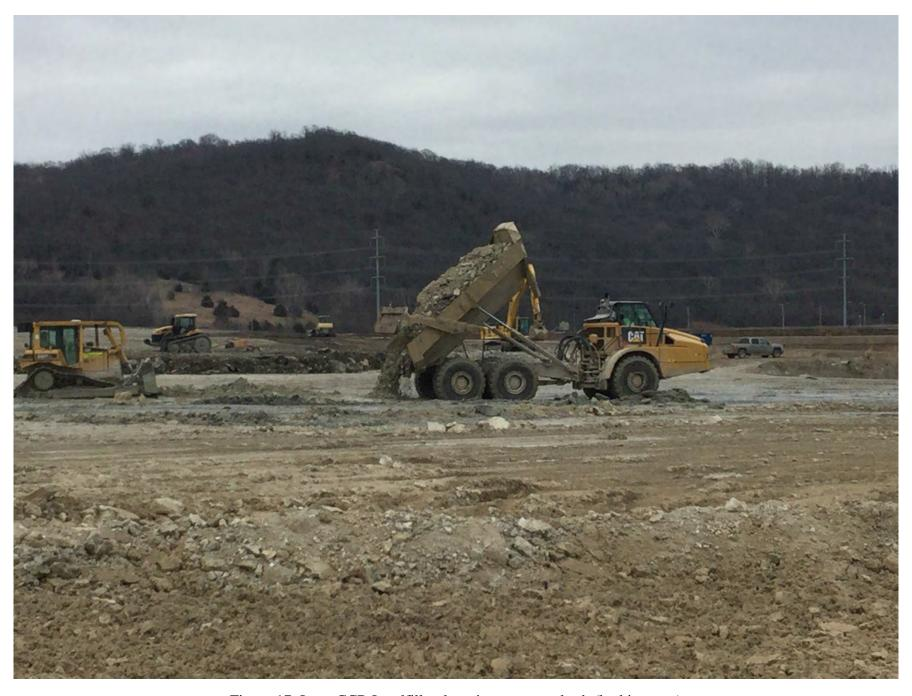
Figure 17: Iatan CCR Landfill – dumping excavated ash (looking east)
