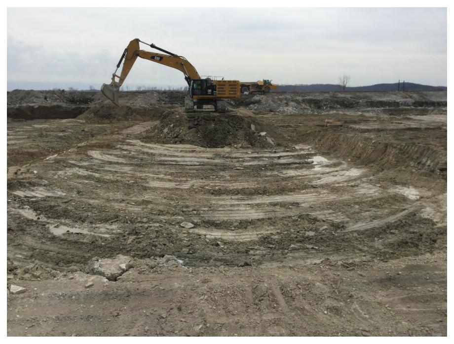
Figure 5: Iatan Ash Impoundment – mechanical excavation from north portion of pond (looking east)
