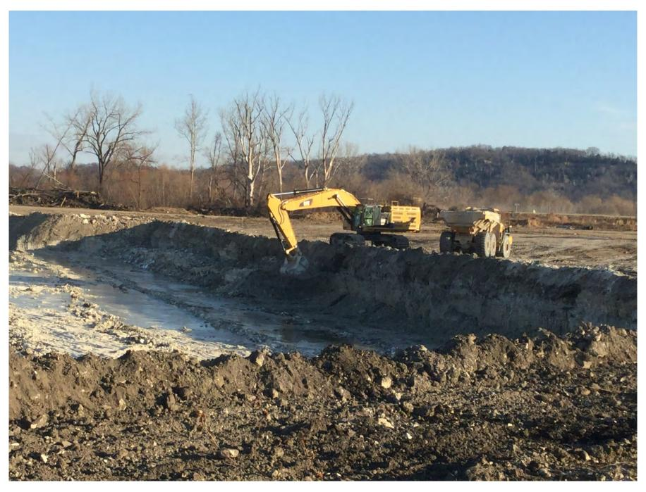
Figure 4: Iatan Ash Impoundment – mechanical excavation from north portion of pond (looking northeast)
