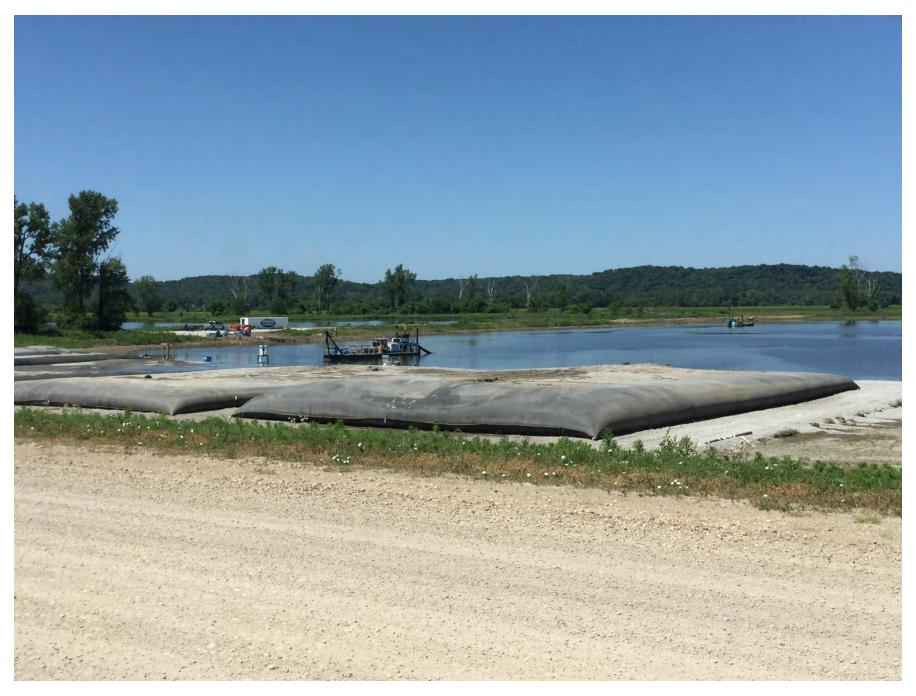
Figure 13: Iatan Ash Impoundment – filled geotextile tubes (east bank looking southwest)
