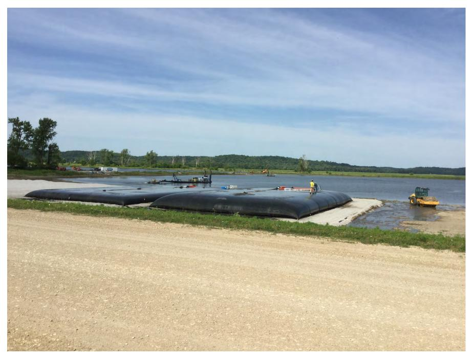
Figure 11: Iatan Ash Impoundment – filling geotextile tubes (east bank looking southwest)
